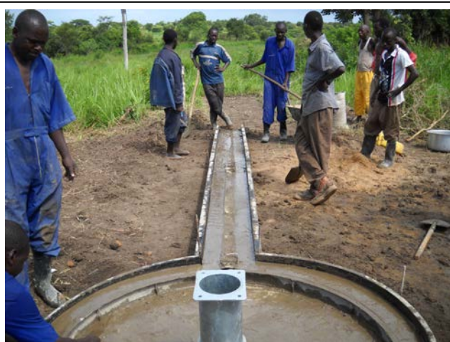
Divine Waters field crew at work casting spillway and cap for new shallow well at Lele-Dam Village. (June 2011).
