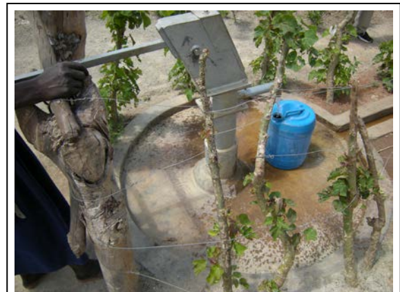
India Mark II Handpump at Bar Odir well where “living fences” were planted to protect the well from animals that could contaminate the area (Nov.2012).
